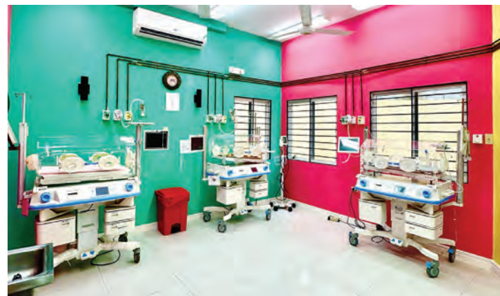
The newly constructed special care nursery at the Annotto Bay Hospital in St. Mary.
