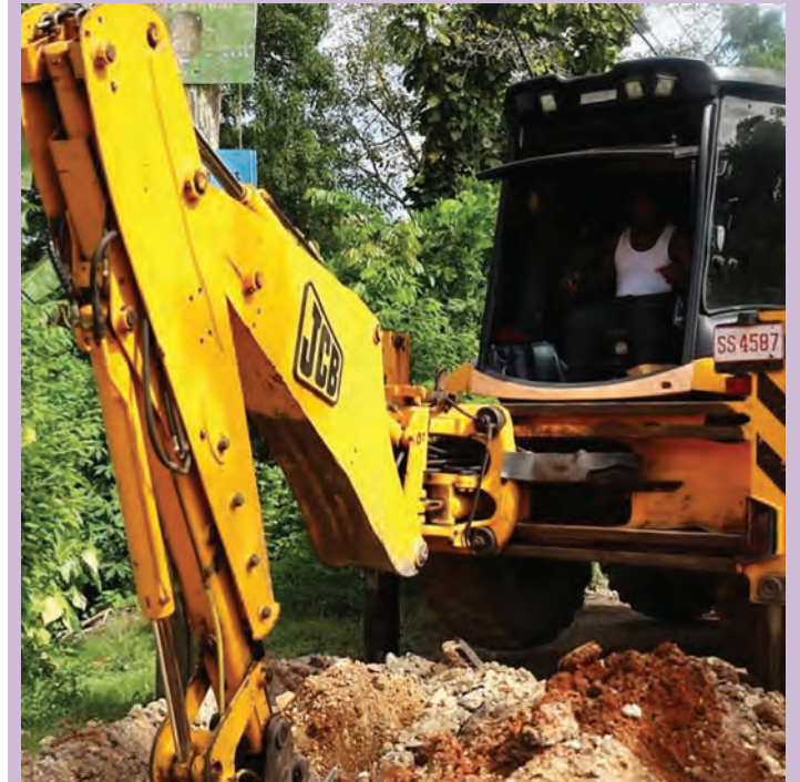
Work underway on the Wentworth Water Supply system in St. Mary.
